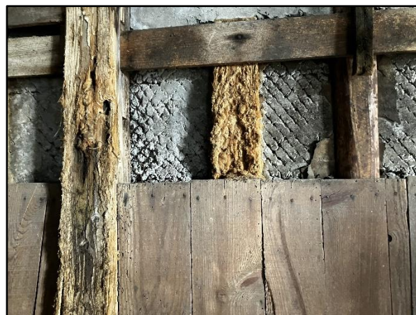
柱の腐朽
